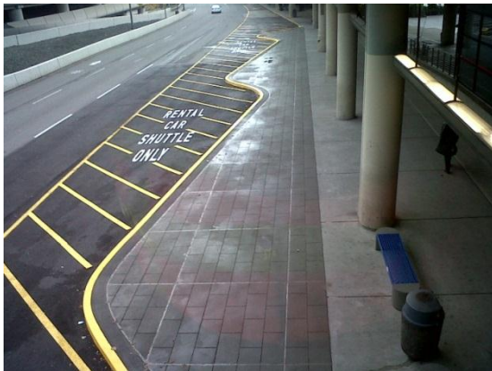
Sidewalk and Shuttle Stop Improvements
