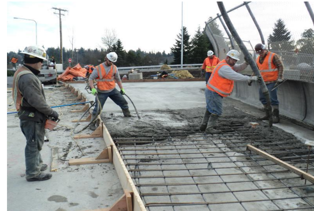
Pouring sidewalk at So. 160 th St Bridge
