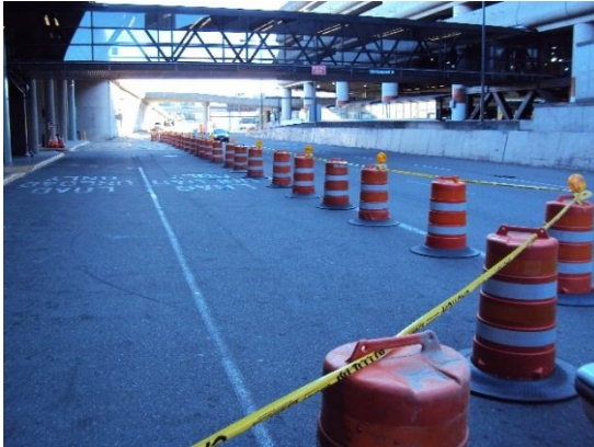
Start of construction
